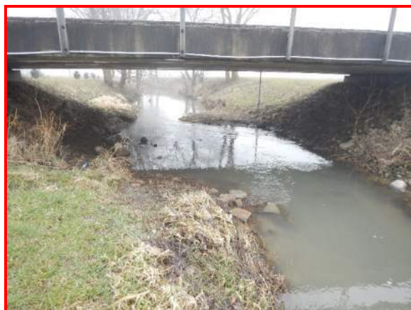
238. Looking south along School Branch, north of CR 750
