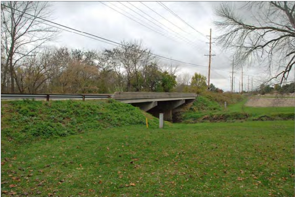
WA-H13_On Cr1000 N E of SR267_Deck and North Elev.JPG
