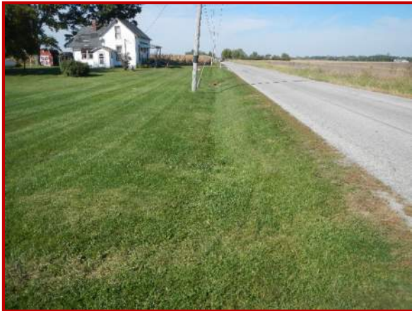
15. Looking north along Hendricks CR 900 E at the roadside ditches
