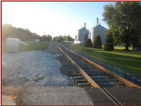
3. Looking southeast along CSX railroad south of Hendricks CR 600 N
