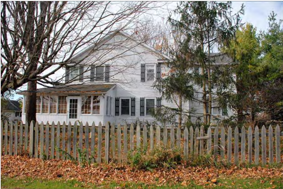
WA-H7_10632 N CR 950 E_E elevation.JPG
