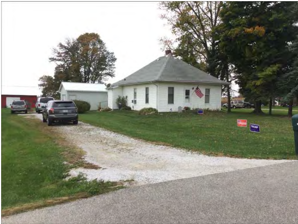
WA-H19_8315 Maloney Road_N and W Elev.JPG
