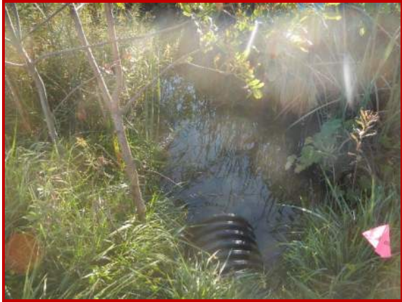
19. Looking northeast at culvert draining into Wetland 6N-B
