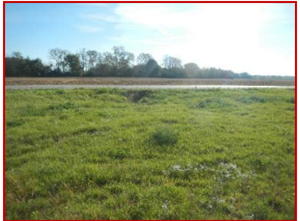
34. Looking east at culvert underneath Hendricks CR 900 E
