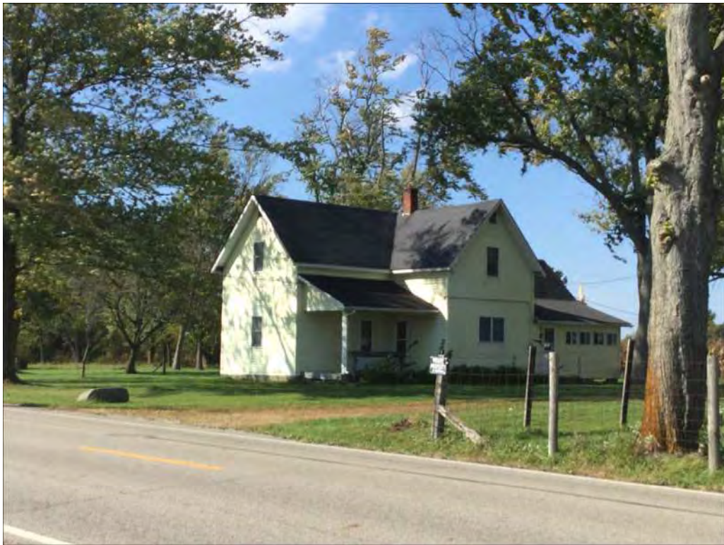
WA-B24_5220 E Whitestown Parkway_House_S and E elevs_Close.JPG
