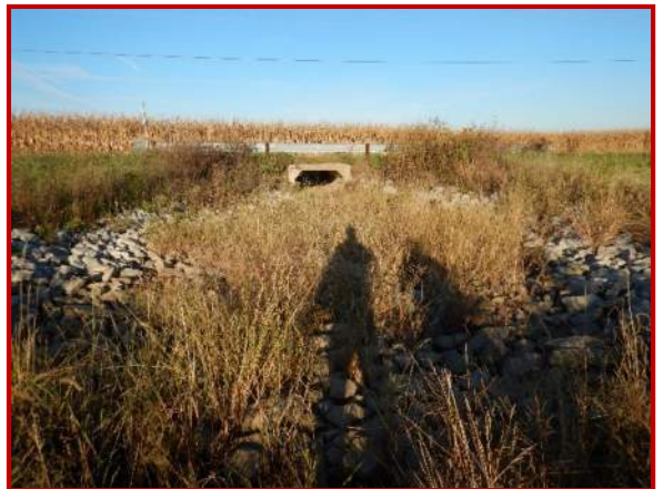
18. Looking west at culvert underneath Hendricks CR 900 E
