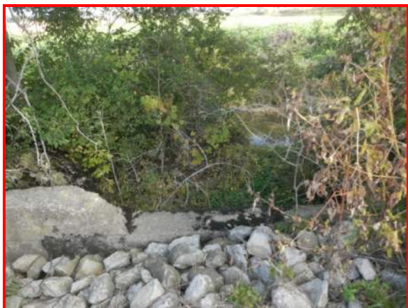
233. Looking northeast at concrete weir, spillway adjacent to White Lick Creek
