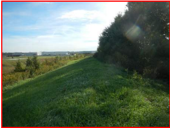
211. Looking east along berm east of SR 267
