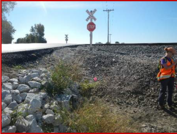
43. Looking south from DP 6N-11 at Wetland 6N-F
