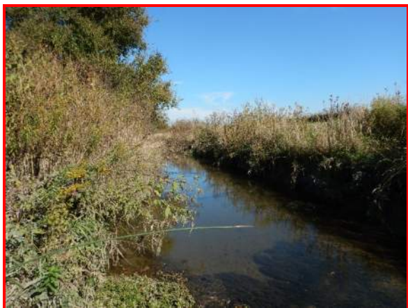
138. Looking northeast along Etter Ditch (upstream)
