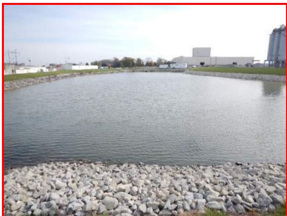
221. Looking east at detention pond along SR 267
