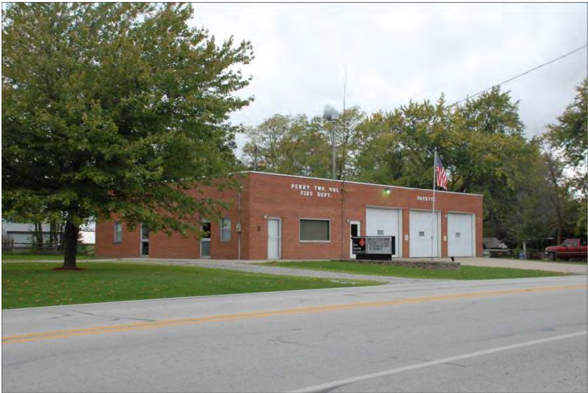
WA-B33_7470 S SR267_Fire Station_S and W Elevs_1964.JPG
