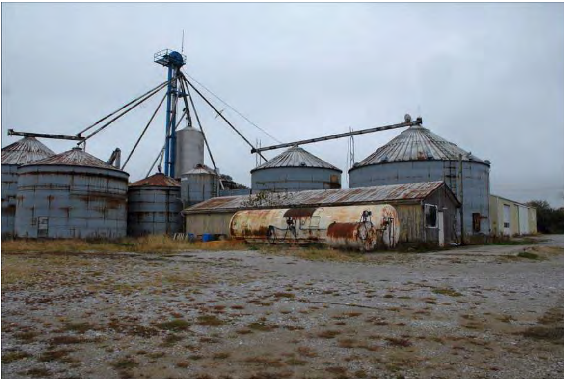
WA-B14_5380 E CR550 S_Old Grain Elevator_Setting_South and West Elevs.JPG
