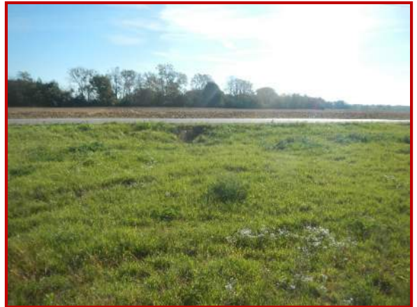
10. Looking east at culvert underneath Hendricks CR 900 E
