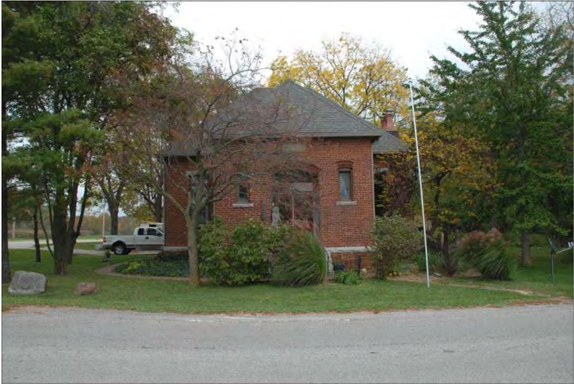
063-117-40004_5985 CR 600 N_Walker School_West Elev.JPG
