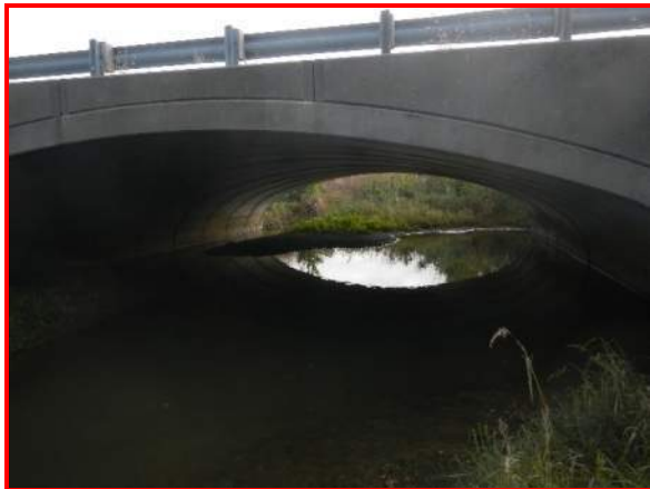
207. Looking east at bridge carrying SR 267 over White Lick Creek (downstream)
