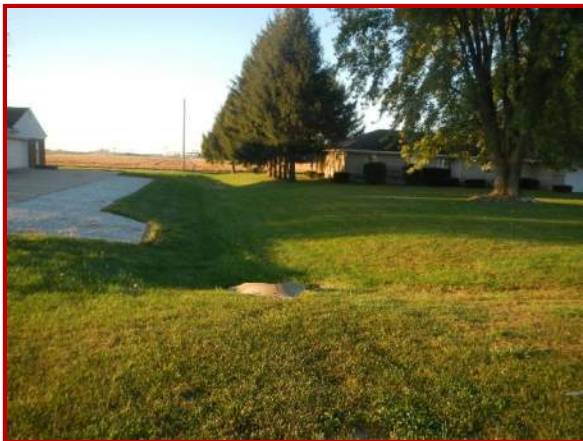
5. Looking south at culvert south of Hendricks CR 600 N
