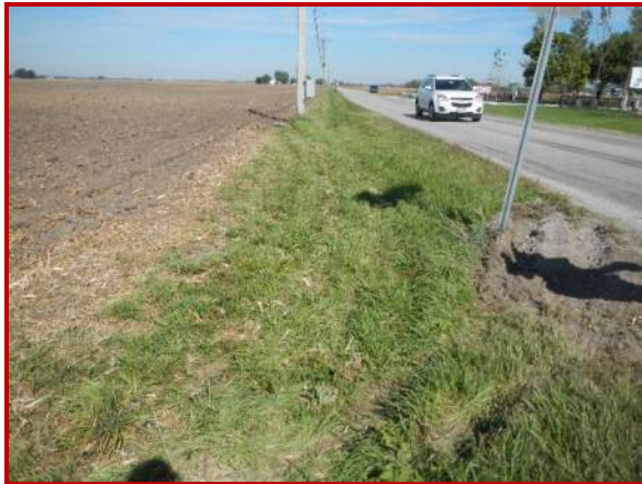
51. Looking north along Hendricks CR 900 E at the roadside ditches
