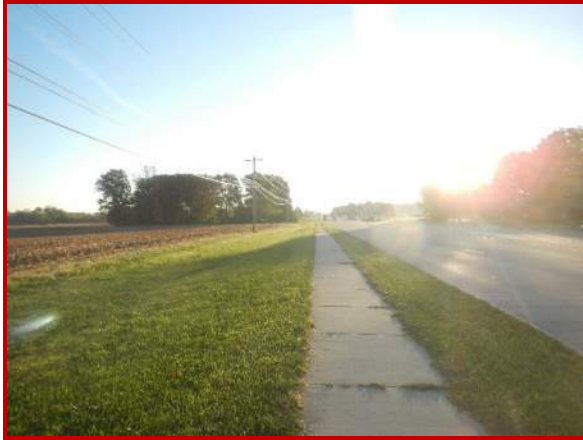
7. Looking east along north side of Hendricks CR 600 N, west of existing Ronald Reagan Parkway's northern terminus
