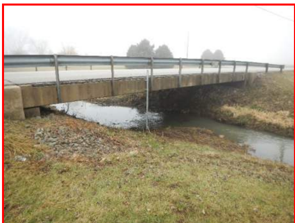
237. Looking northeast at bridge carrying CR 750 over School Branch
