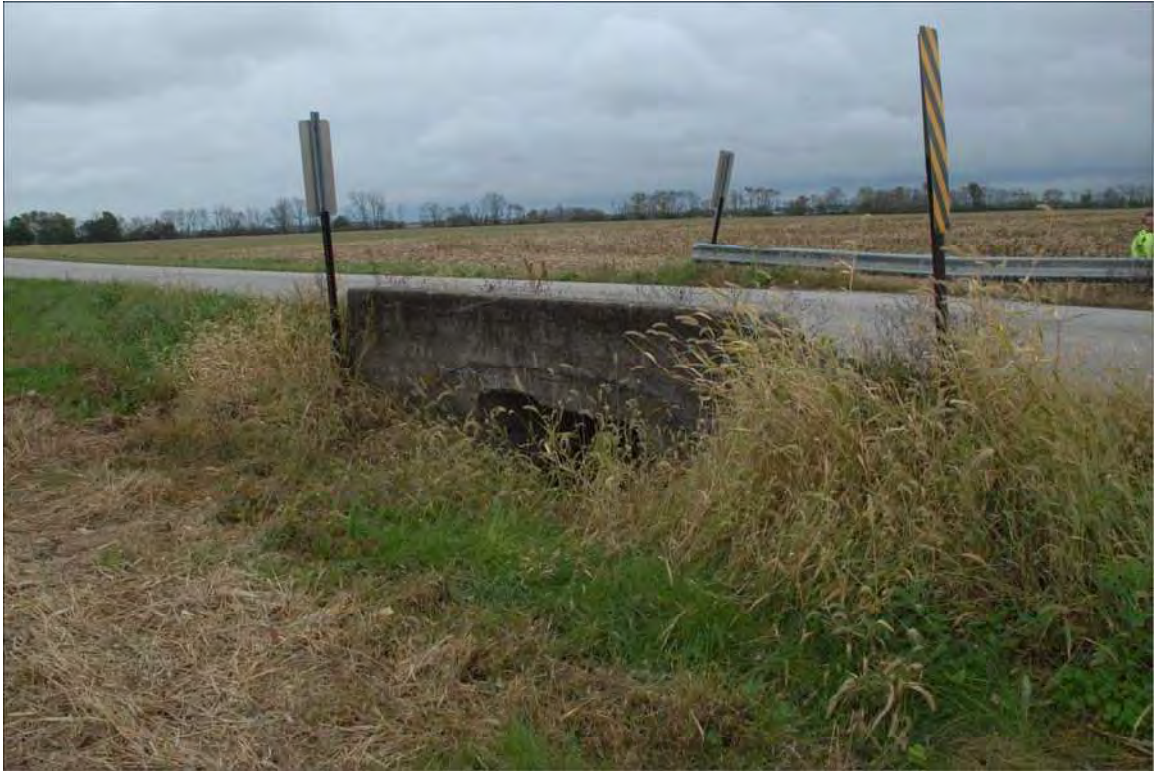
WA-H21_Culvert_S Elev_East of CR900 E.JPG
