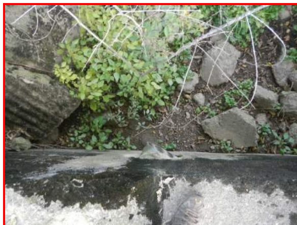
234. Looking down at tile outlet into White Lick Creek
