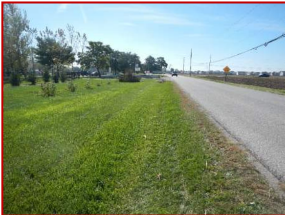
11. Looking south along Hendricks CR 900 E at the roadside ditches
