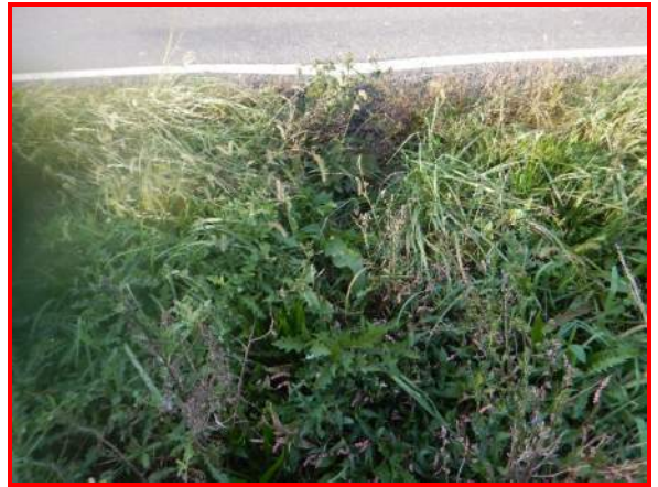
92. Looking north at pipe outfall underneath Hendricks CR 1000 N
