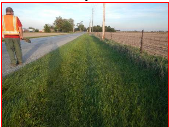
191. Looking east along south side Boone CR 550 S west of SR 267
