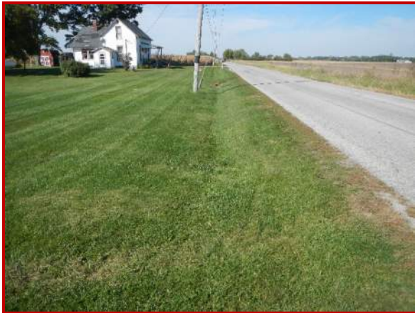
57. Looking north along Hendricks CR 900 E at the roadside ditches
