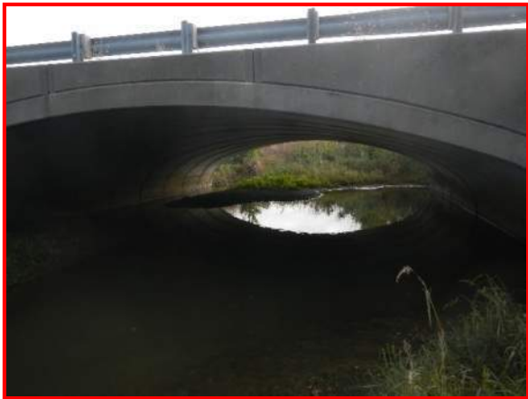
51. Looking east at bridge carrying SR 267 over White Lick Creek (downstream)
