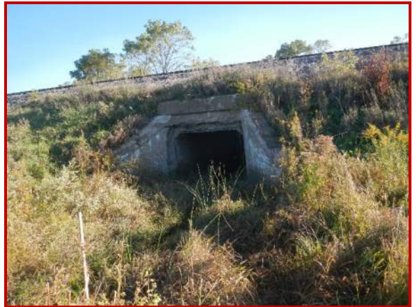
22. Looking northeast at bridge carrying UNT 1 under CSX Railroad
