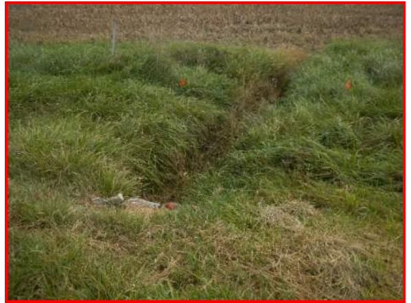
194. Looking east at culvert underneath SR 267
