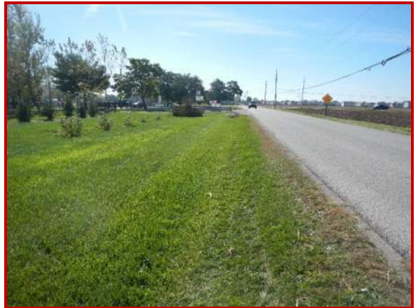
52. Looking south along Hendricks CR 900 E at the roadside ditches
