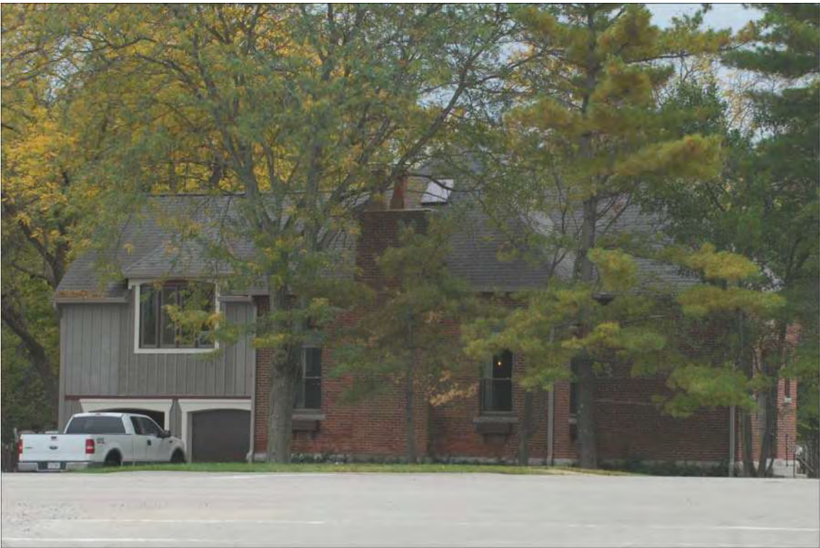
063-117-40004_5985 N CR1000 E_Walker School.JPG
