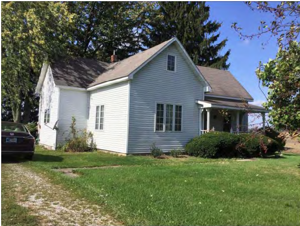
WA-B16_5720 S SR267_E Elev_Looking W.JPG
