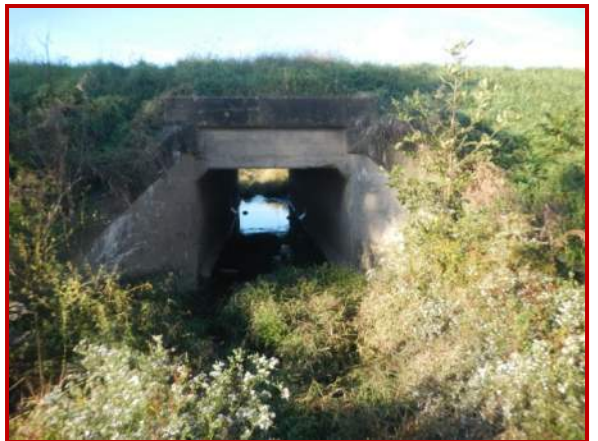
24. Looking southwest at bridge carrying UNT 1 under CSX Railroad
