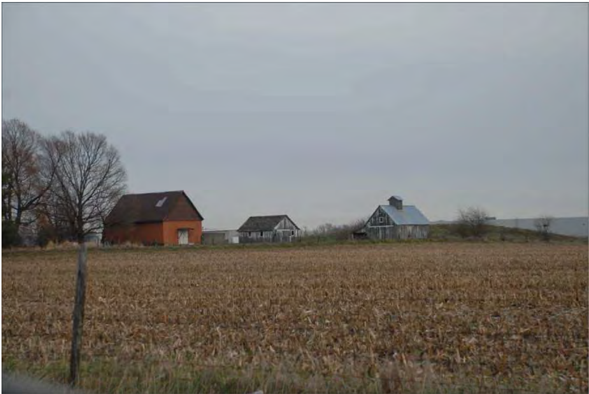
WA-B9_4955 SR 267_Outbuildings South and West Elev_Zoom.JPG
