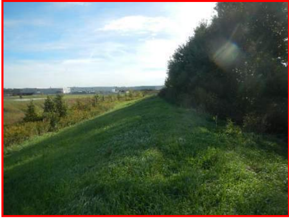
49. Looking east along berm east of SR 267
