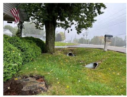
Photo 4. Looking south at two unnumbered corrugated metal pipe culverts in upland area of Investigated Area.
