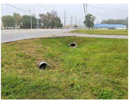
Photo 5. Looking north at two unnumbered corrugated metal pipe culverts in Investigated Area.
