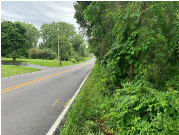
Photo 7. Looking west along CR 1100 N.
