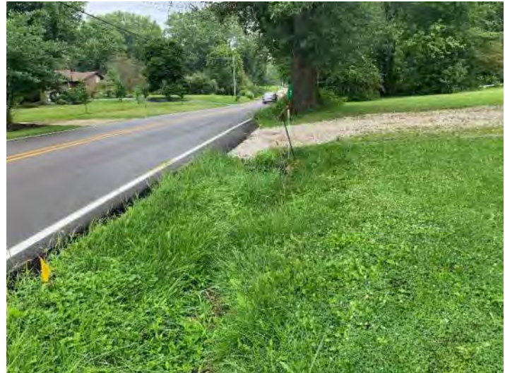
Photo 52. Looking west along CR 1100 N.
