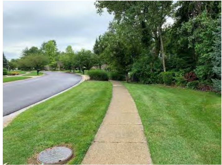
Photo 96. Looking southwest along Laurel Creek Drive on the existing sidewalk.
